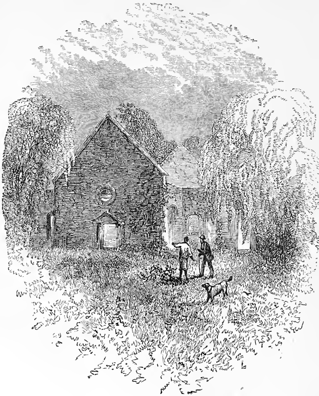
WALLS OF ST. JOHN'S CHURCH.
